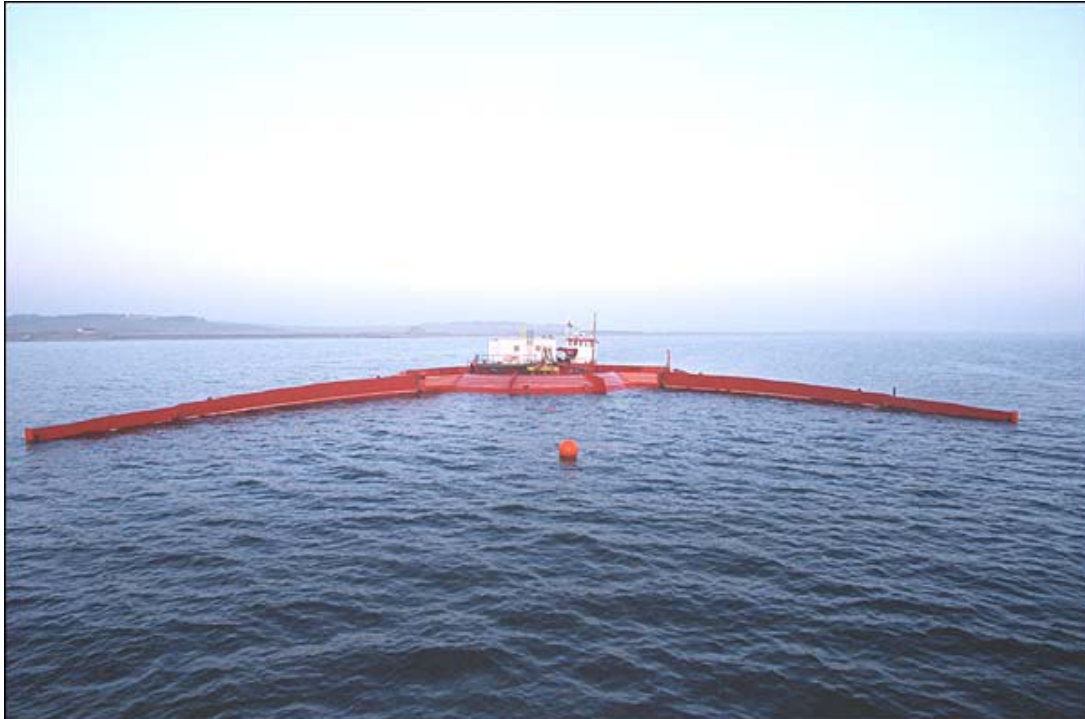
Figure 9: Wave Dragon (overtopper) prototype showing tapered channel and ramp © Wavedragon ( http://www.wavedragon.net , 2010)
