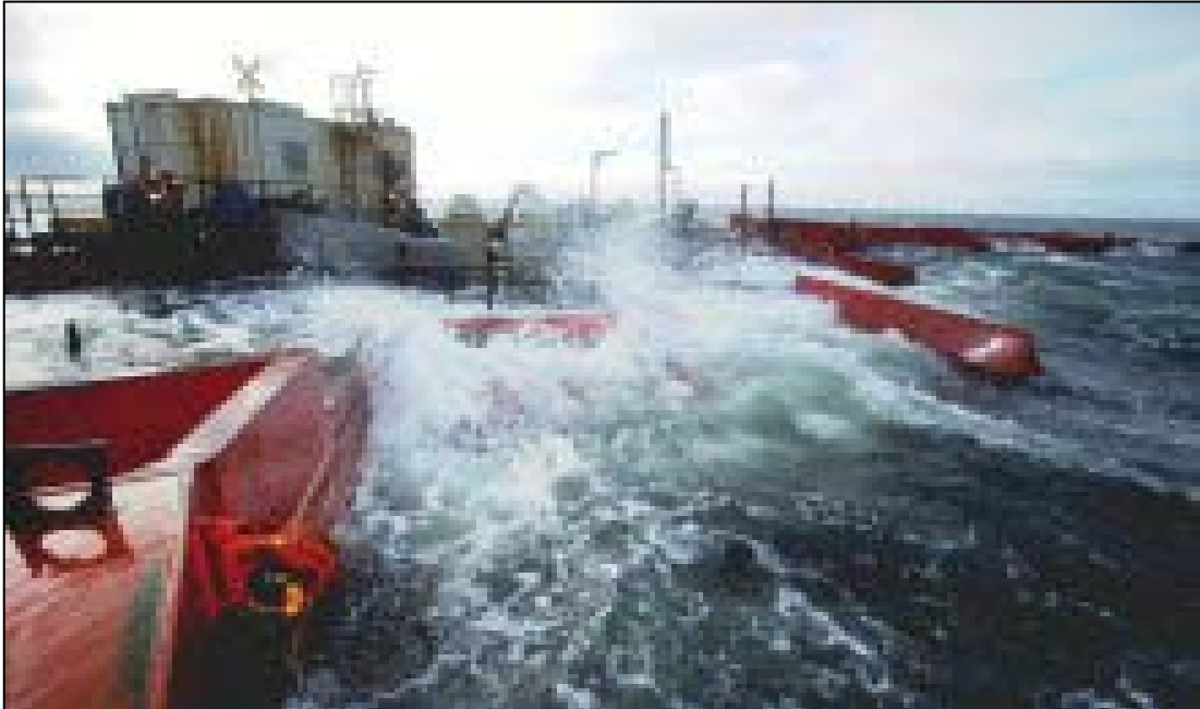
Figure 8: Wave Dragon (overtopper) prototype with an overtopping wave © Wavedragon ( http://www.wavedragon.net , 2010)
